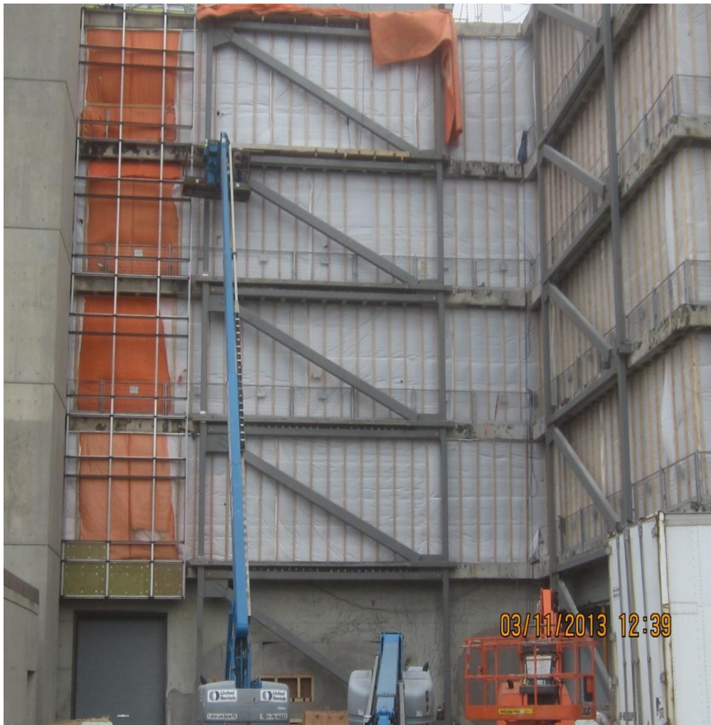
Figure 6. West wall of Sawyer Building Mod 5 at RMC showing seismic upgrades
